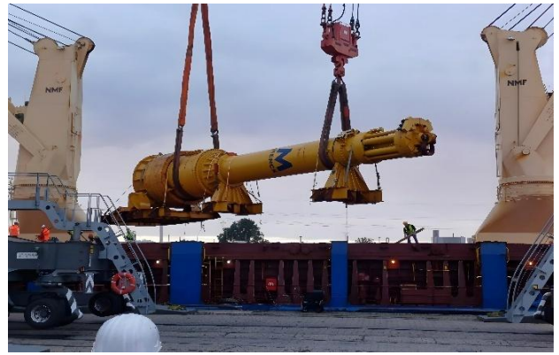
Door to Door Handling of 150 Ton Hammer - Hazira Port to Malaysia
