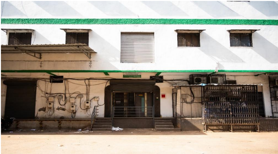
Outer view of the warehouse facility
