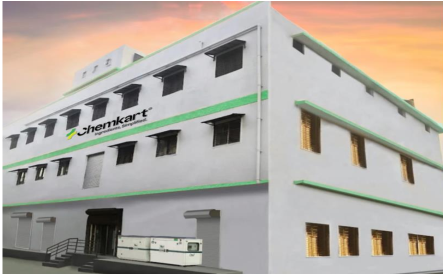
Full Image of Warehouse
