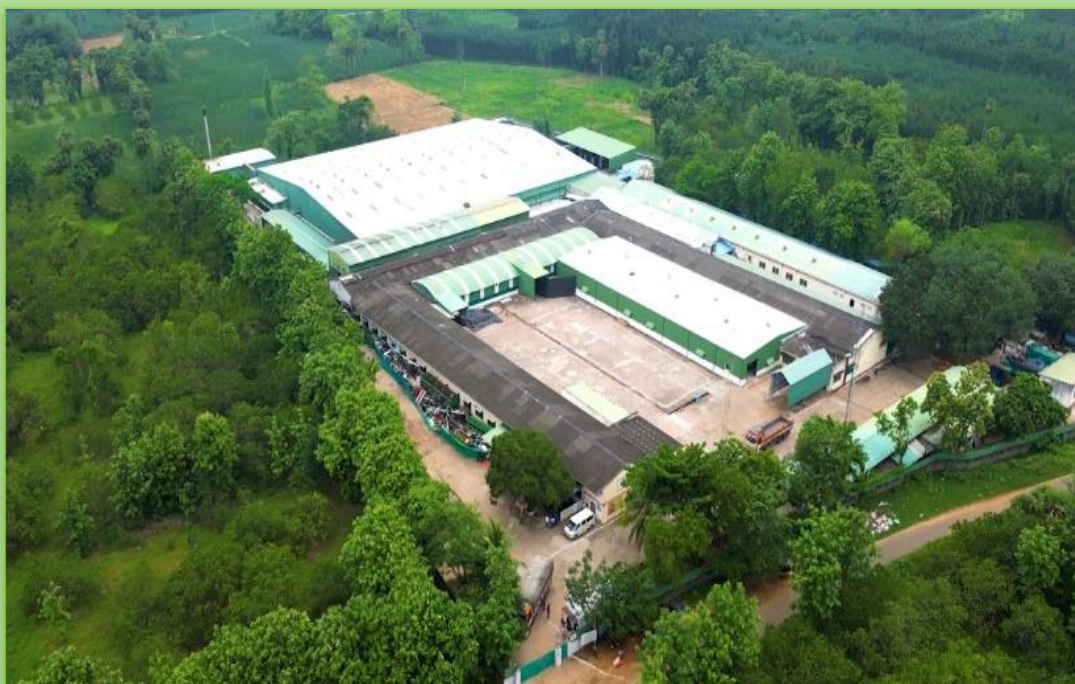
Cashew Processing Plant
