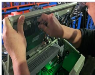
4. PLC Control System
